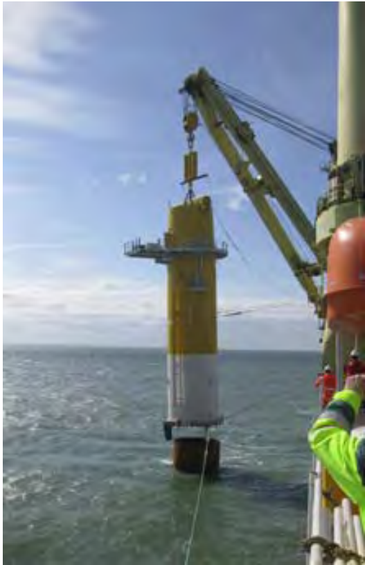
Figure 5.4. Transition Piece Being Placed over Monopile
