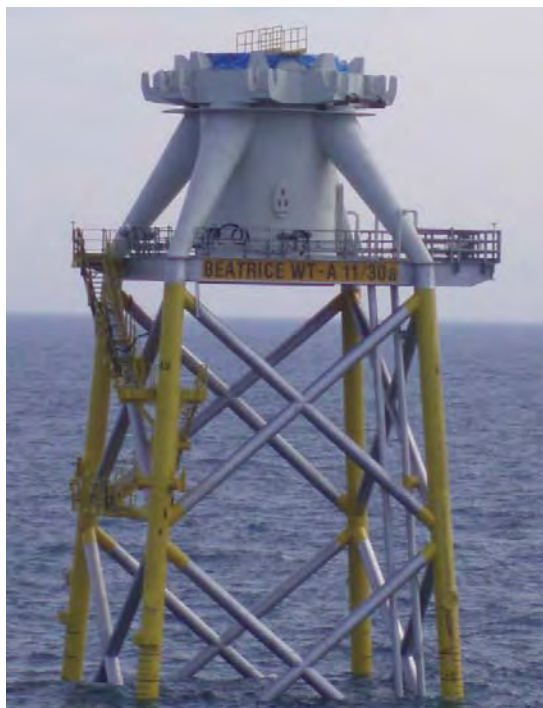
Figure 5.6. Jacket and Transition Piece at Beatrice
