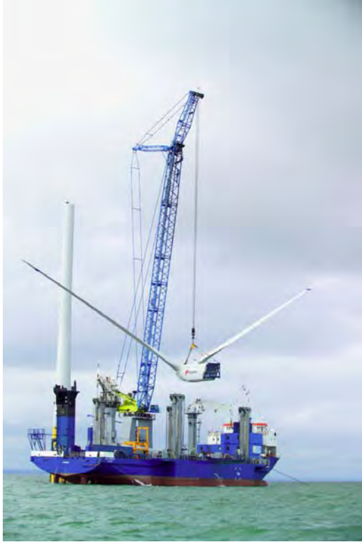
Figure 5.11. Nacelle and Blades in the Bunny Ear Configuration at Kentish Flats
