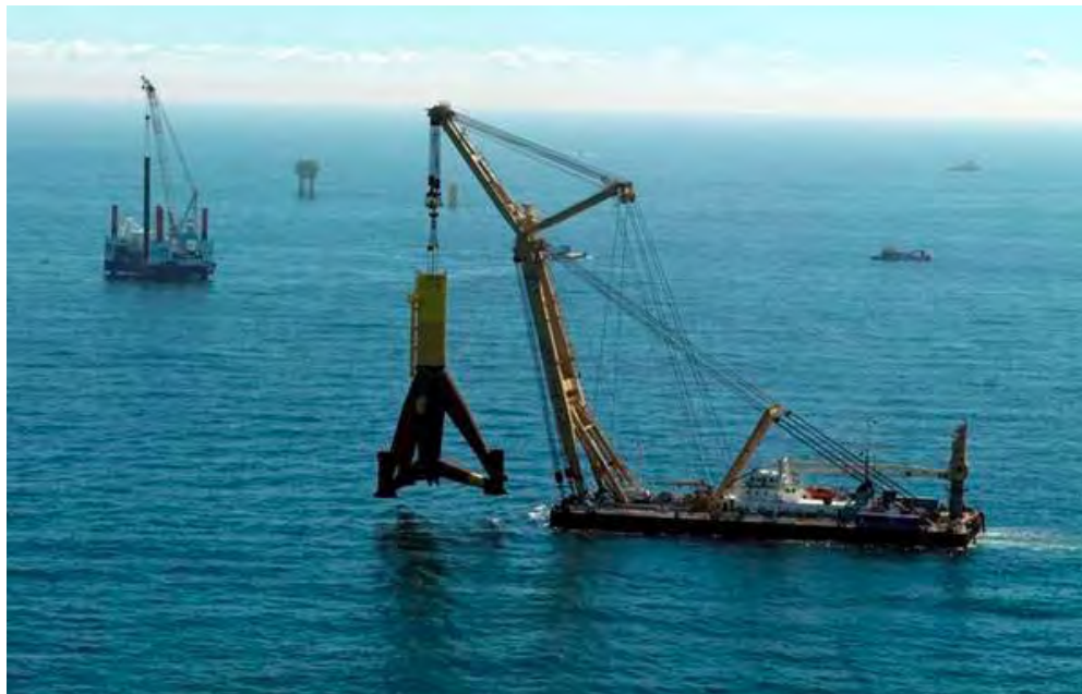
Figure 2.4. The Taklift 4 Placing a Tripod Foundation at Alpha Ventus Source: Alpha Ventus 2010
