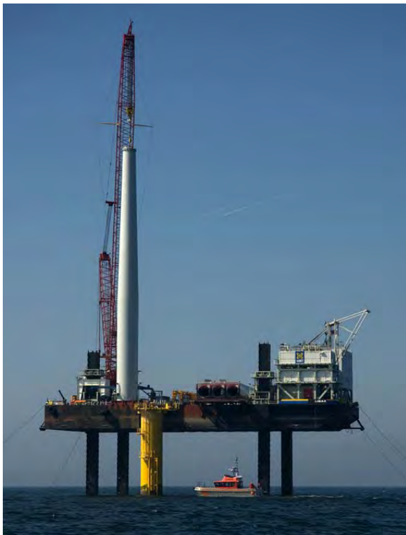
Figure 5.9. Lifting a Fully Assembled Tower onto a Transition Piece at Rhyl Flats Source: RWE npower 2010
