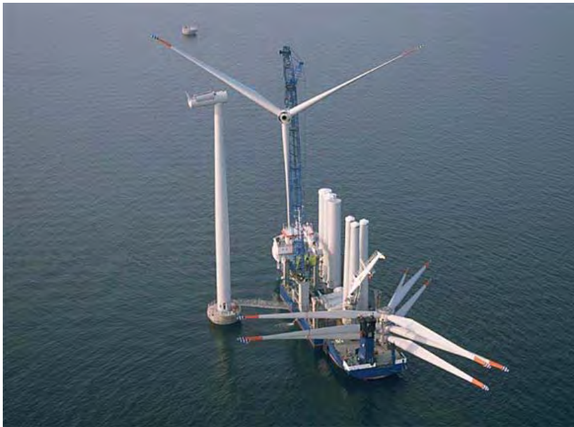
Figure 2.12. An Assembled Rotor Being Lifted onto a Nacelle at Nysted
