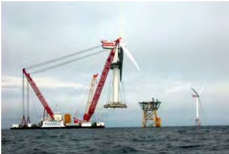
Figure 6.5. The Heavy Lift Vessel Rambiz Installing a Turbine at the Beatrice Project
