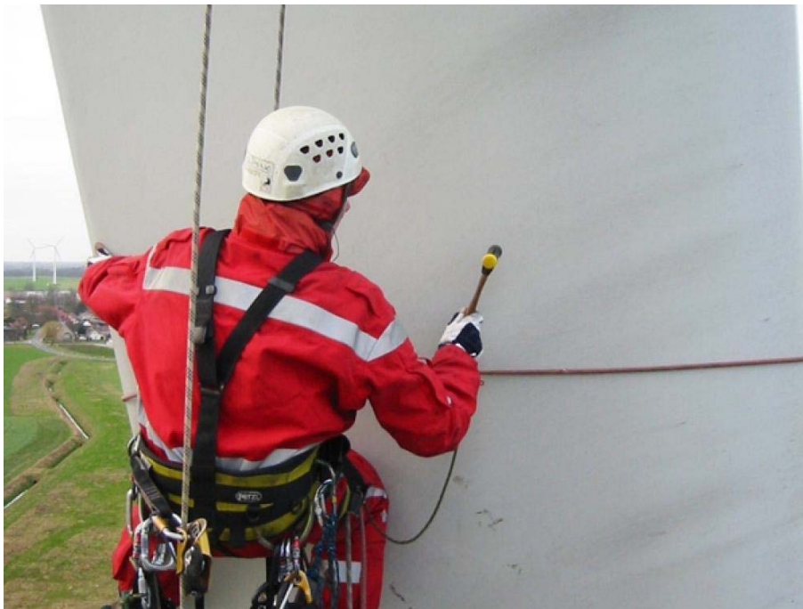
Figure 1 – Rotor Blade Inspection via Rope Access
