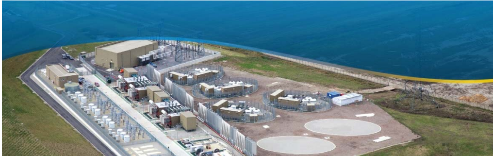
Figure 26 – London Array Onshore Substation 114
