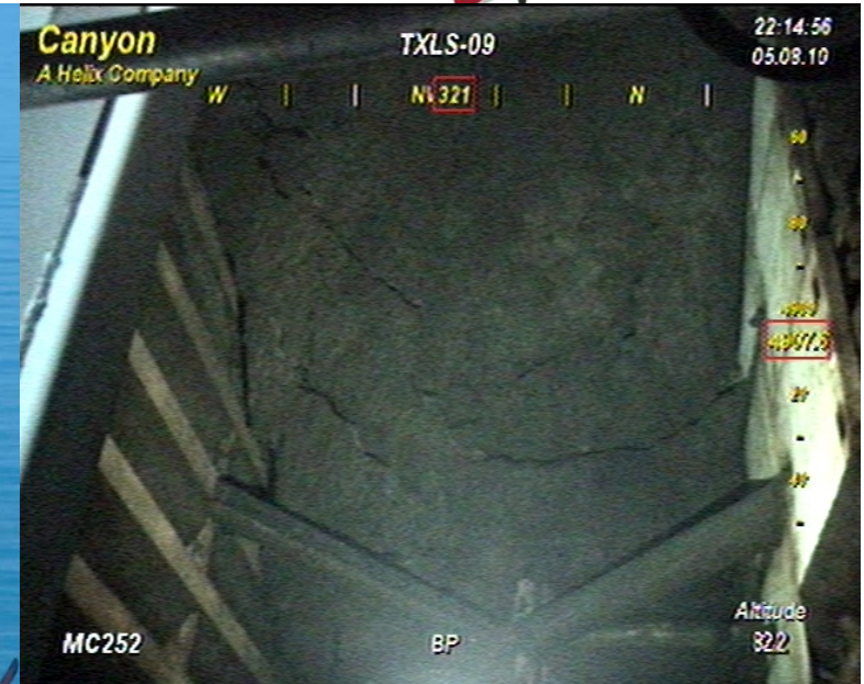
Hydrate in the containment dome
