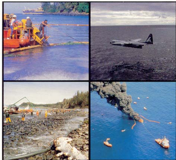
Top left: mechanical containment and recovery; top right: dispersant application; bottom left: shoreline cleanup; bottom right: in-situ burning.
