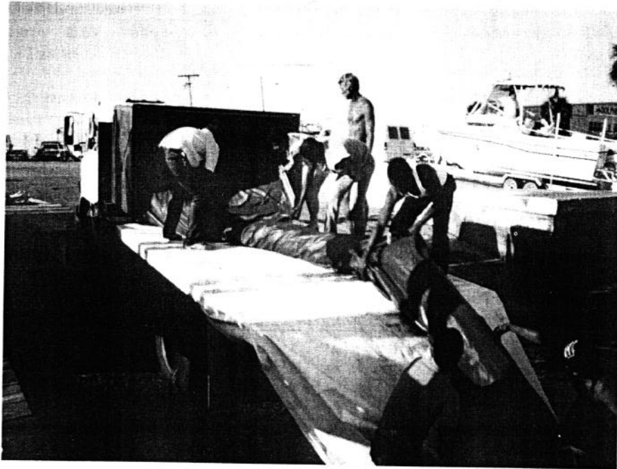
FIGURE 9 WORKERS DEPLOYING FIRE BOOM FROM FLATBED TRUCK INTO THE HARBOR
