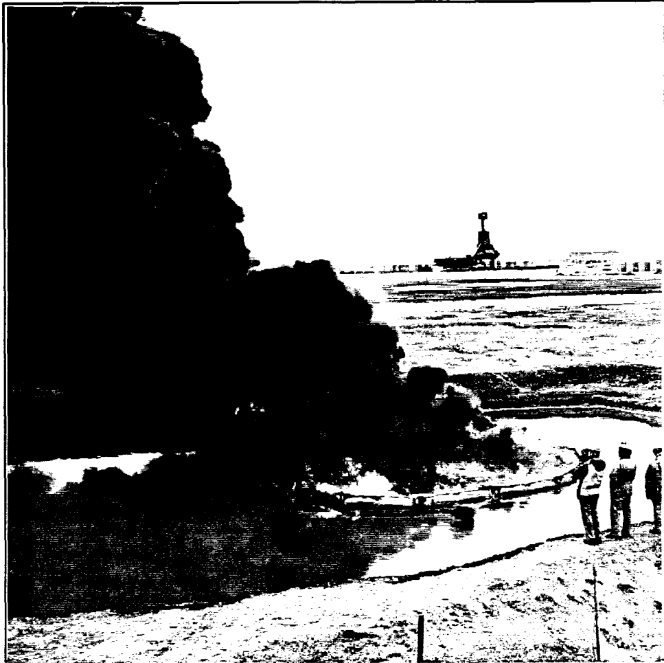
Figure 65 Burn area returned to 100% - note oil loss from fire boom
